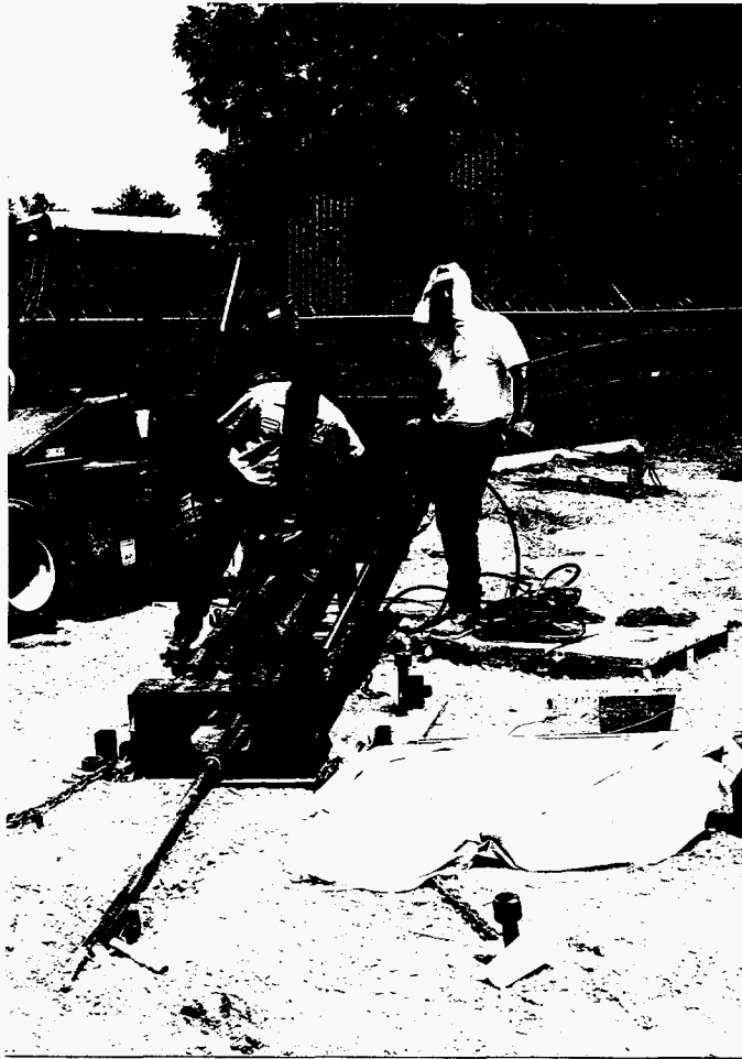
Figure 35. Sub-horizontal field test set-up.
