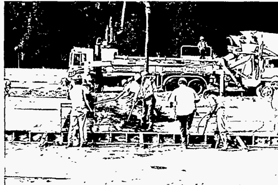
Figure 3.2 C-745-S Cylinder Yard Construction
