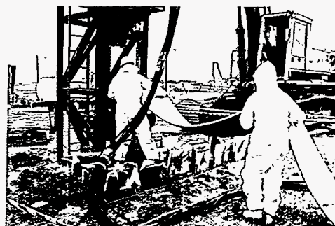
Figure 9.12 Installation of the Lasagna® Demonstration
