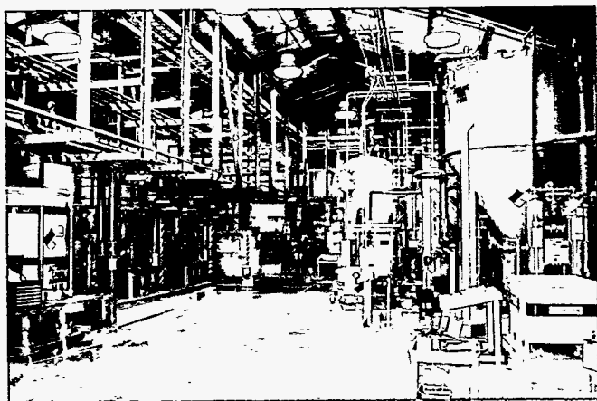
Figure 4. Northwest treatment facility.
