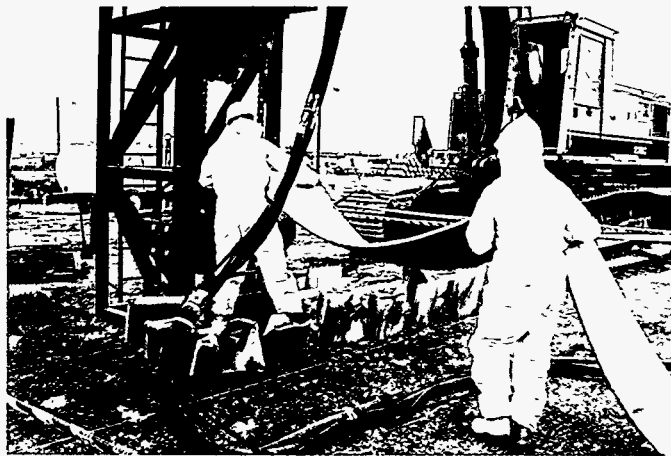
Figure 6. Lasagna® demonstration project installation.
