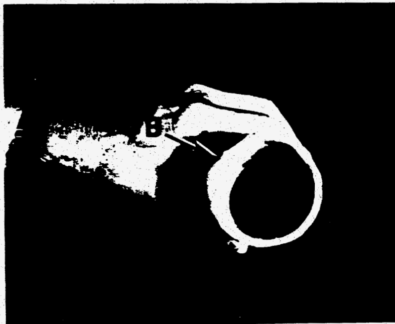
Figure 8. Cross sectional view of pipe in Figure 7 shows pit depth is approximately equal to full wall thickness.
