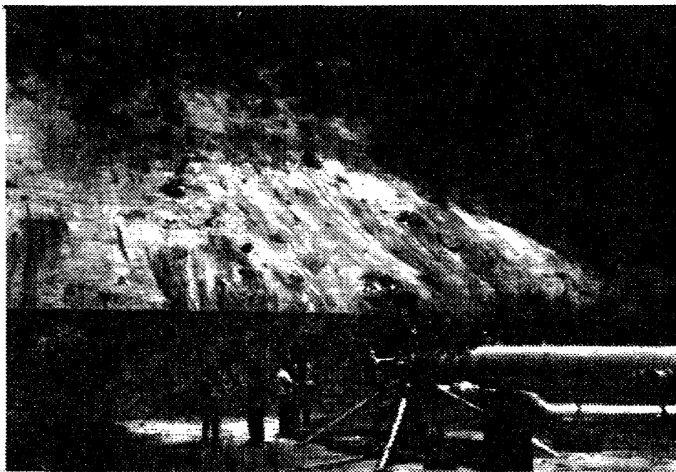
Fig. 4: Photo of well TR-2 showing grouted slope, Berlin geothermal field, El Salvador. The grout did not prevent continued ground cracking and other "creep" phenomena in the landslide encompassing the well.
