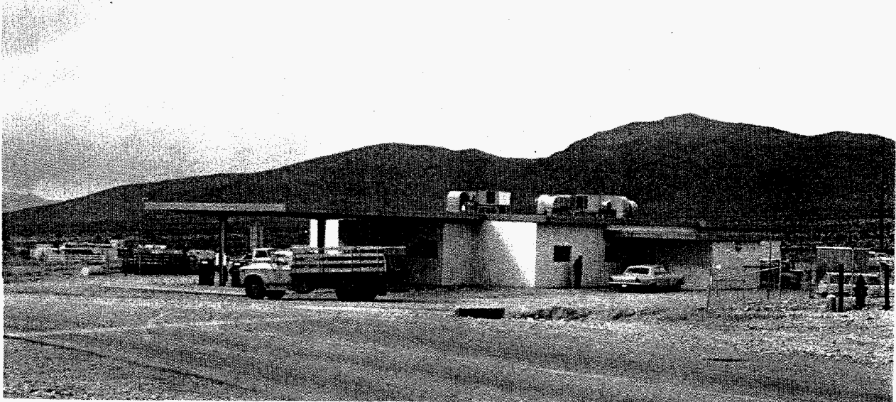
Fig. B-1. Typical Mercury masonry construction.
