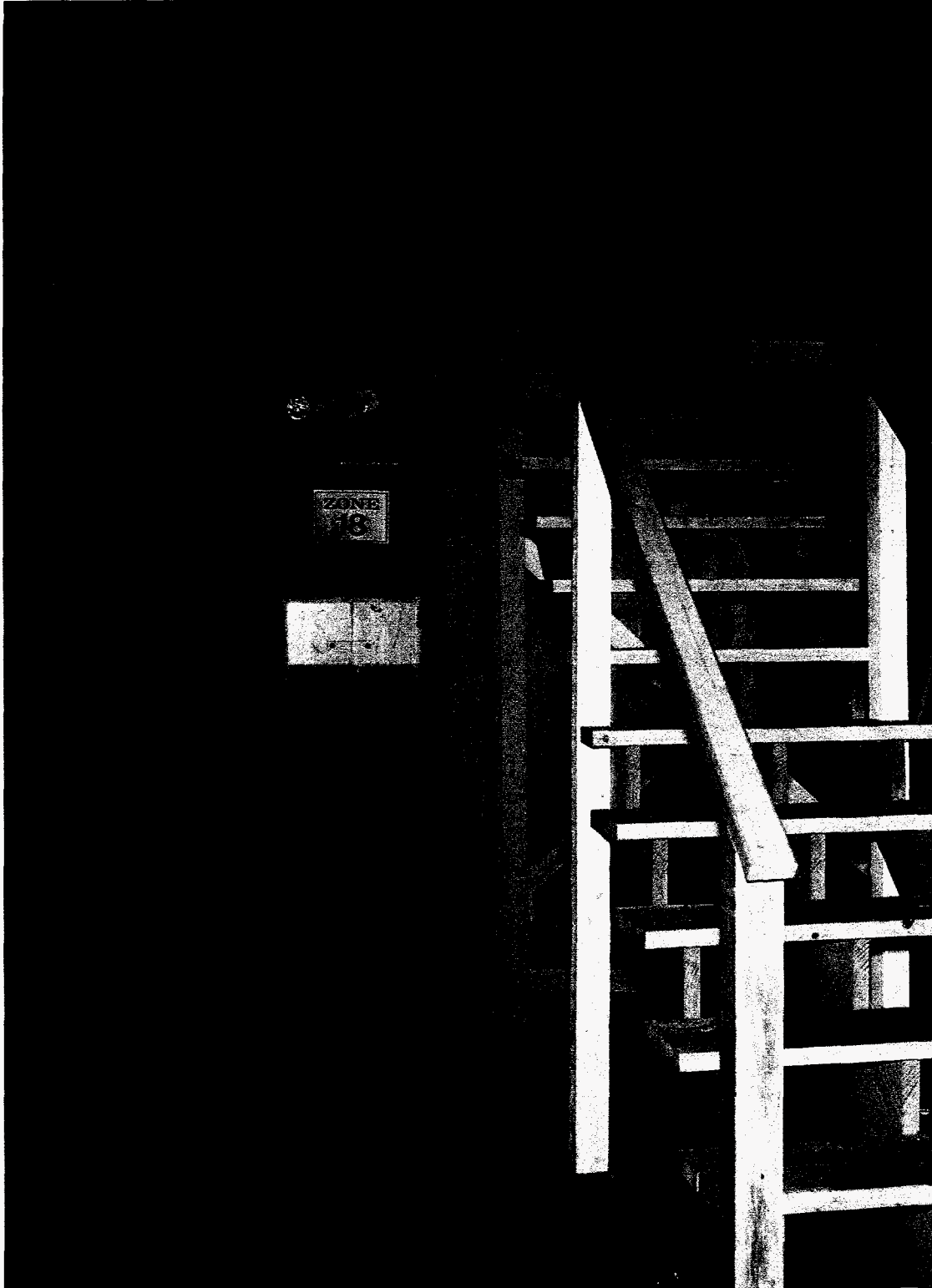
Fig. A.4. Safety upgrades. Safety upgrades for the exit and emergency lights were completed. Stairways were added at the end of elevated work stations to reduce the traveling distance to emergency exits.
