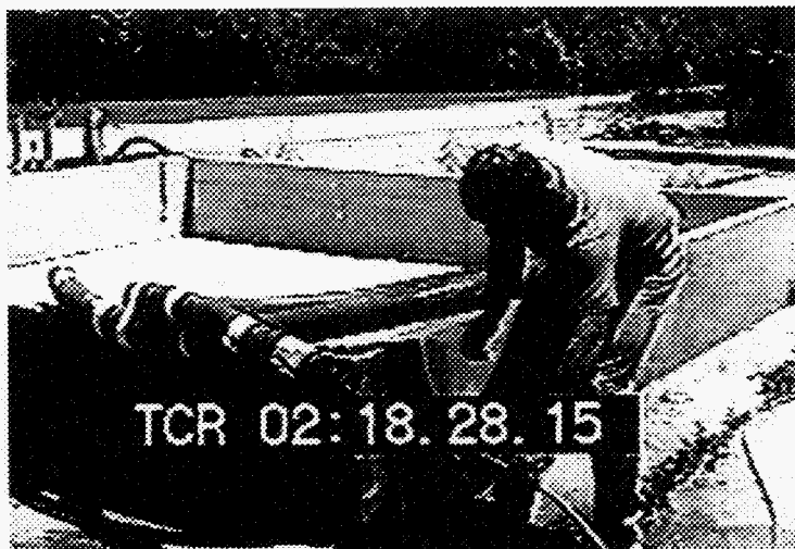
Photograph 20. Insertion of Water Lance into Plugged Line
