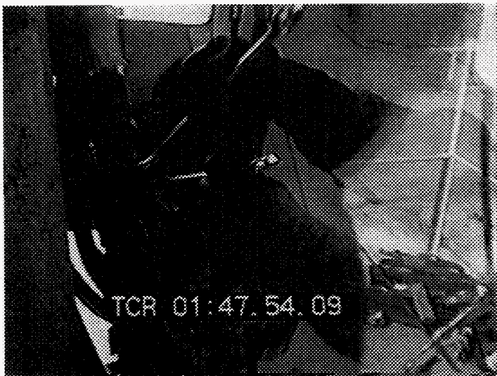
Photograph 33. Mechanics Replacing Hydraulic Lines
