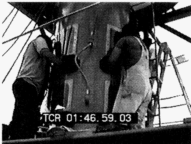
Photograph 31. Mechanics Performing Maintenance on TracPump™ in DCCV
