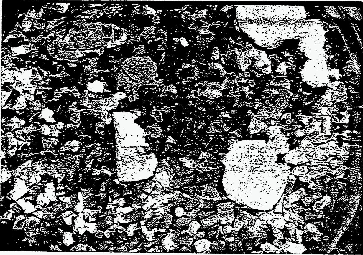
Figure 15. DUCRETE made with \text{UO}_2 aggregate after exposure to 250^\circ\text{C} for 14 days. The DUCRETE completely disintegrated although the \text{UO}_2 pellets are intact. The pellets had a dusty appearance.
