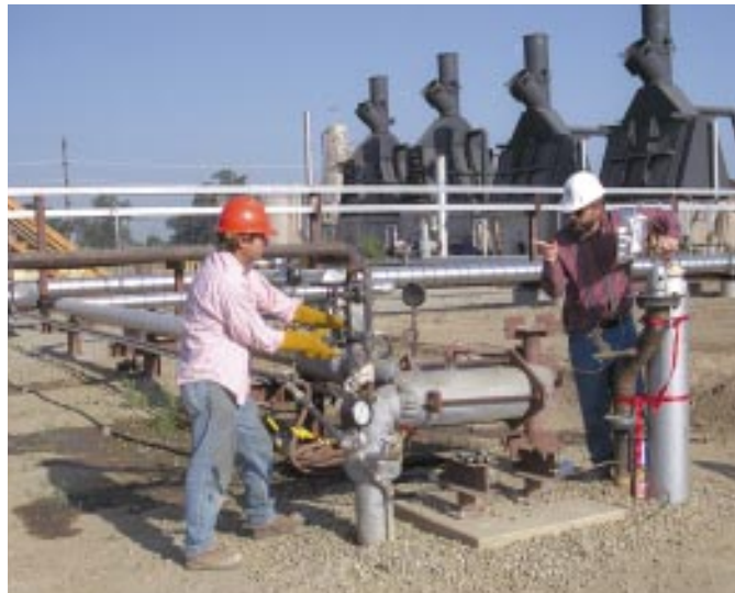
Figure 5. Livermore physicist Bryant Hudson (right), who has developed several methods for monitoring groundwater with noble-gas tracers, adjusts the gas flow with mechanical technician Allen Elsholz. Tanks of noble gases are nearby, and boilers are in the background.
