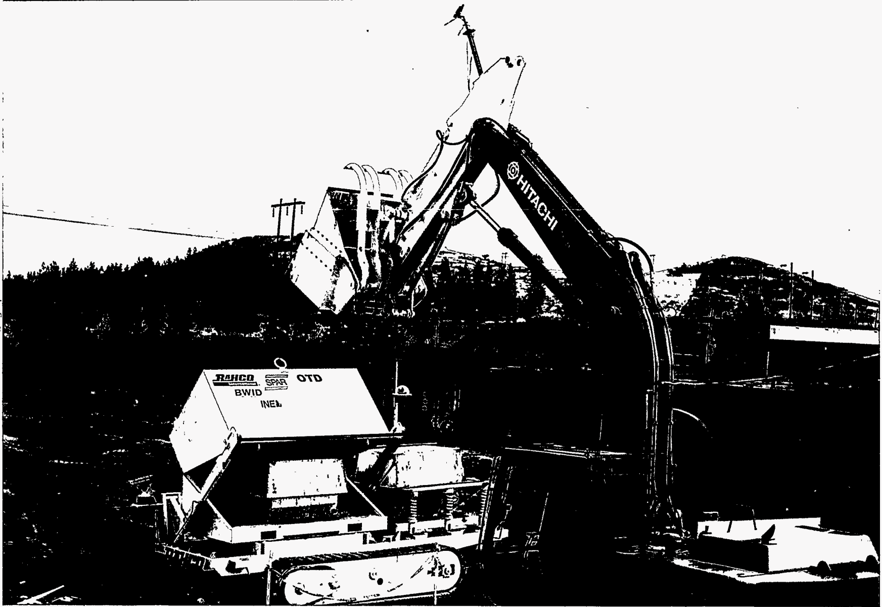
Figure 8. The Hitachi EX-200LC REMEX was modified to a front shovel configuration for belowgrade excavation (INEL 94-1187-28-4).
