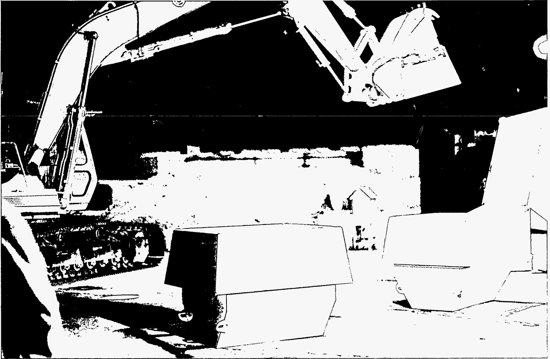
Figure 10. The Phase I test was performed inside a building where wind would not affect the dust and rare earth tracer measurements (INEL 94-1187-20-13A).
