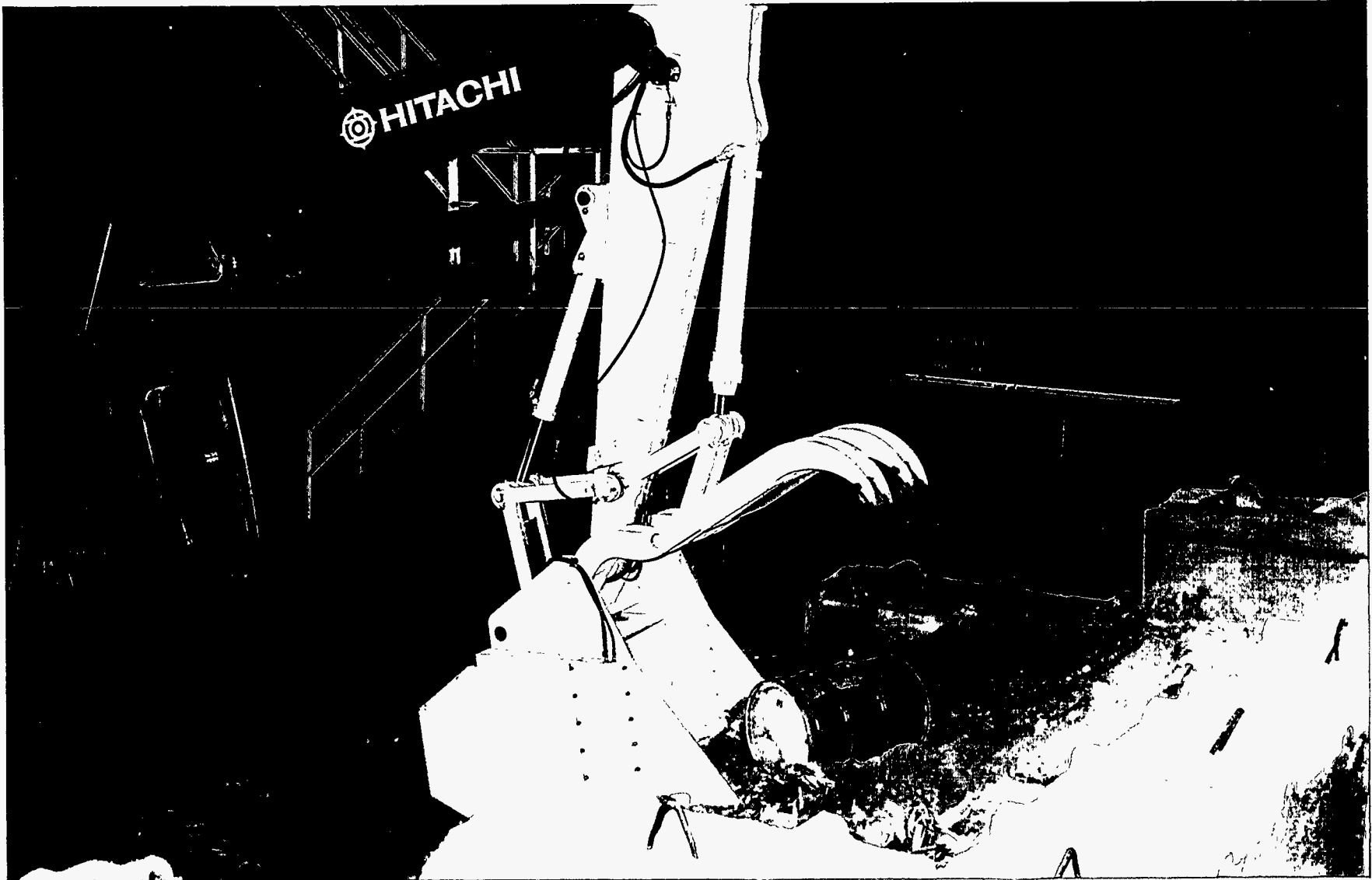
Figure 25. The IEE was flexible in its ability to pick up drums in two ways: either by depositing the drums into the attached ITM (as shown) or by using the bucket and thumb to pick up the drum and then deposit it into a detached ITM. The drums were filled with dry Portland cement (INEL 94-1187-29-4).
