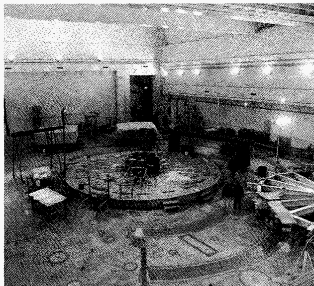
Figure 3. The Tokamak Fusion Test Reactor Test Cell in 1981 prior to machine installation. (PPPL#81E1297)
