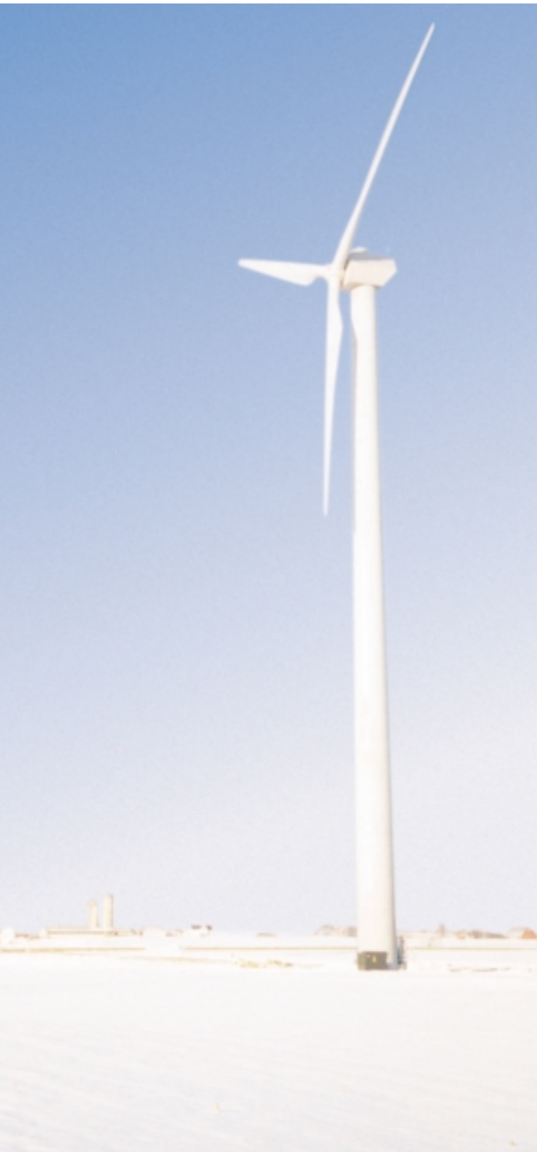
A group of Wisconsin utilities purchased two wind turbines optimized for operation in low wind speeds. The annual average wind speed at the site is 13.7 miles per hour (6.1 meters per second).
