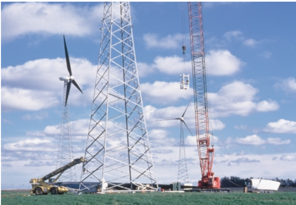
When completed, the 193-megawatt wind power project near Alta, Iowa, will be the single largest wind project in the world. The Zond Z-750 kW Series wind turbines, developed by Zond Energy Systems, Inc., will output enough power for 71,000 average Midwestern homes. Two large utilities will purchase the power to meet a state mandate.
