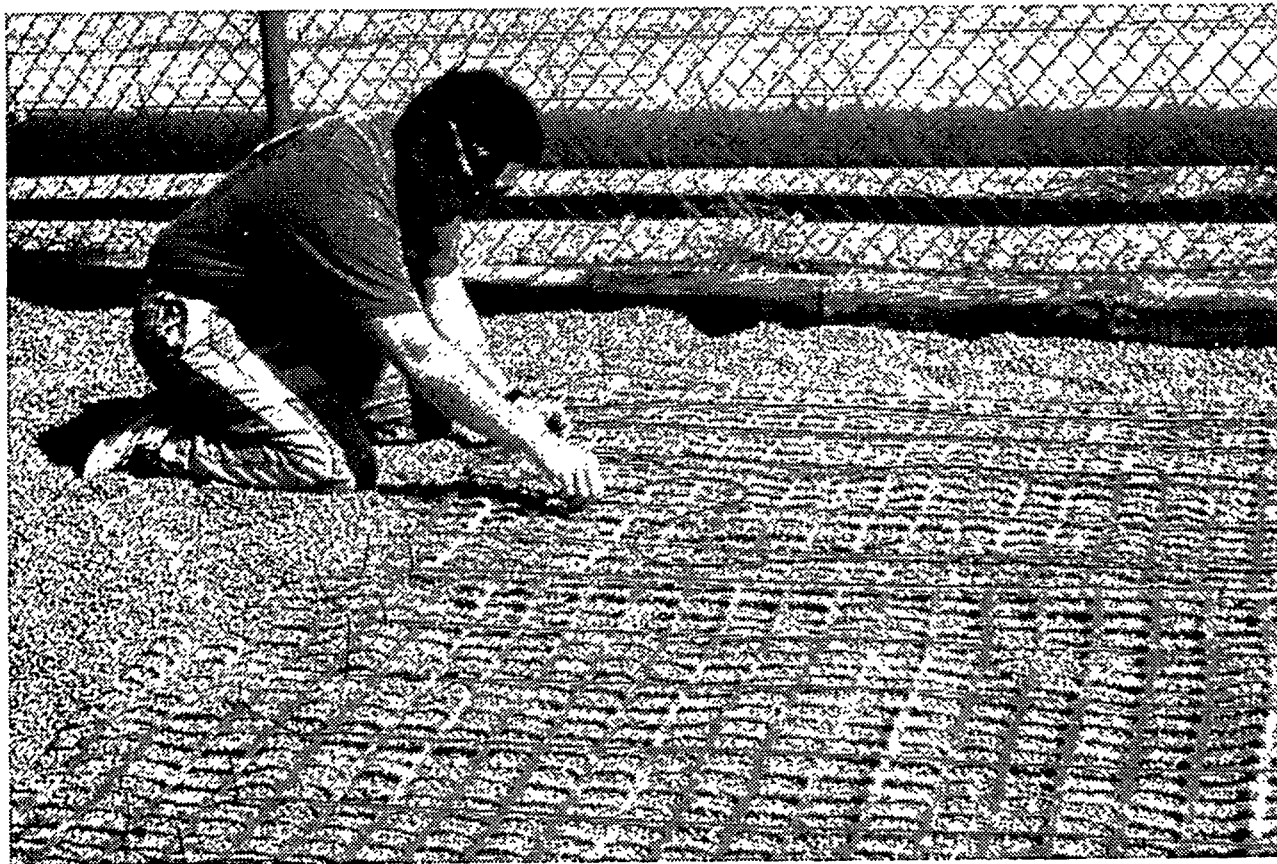
Figure 5-11. Buried installation of fiber-optic intrusion detection system
