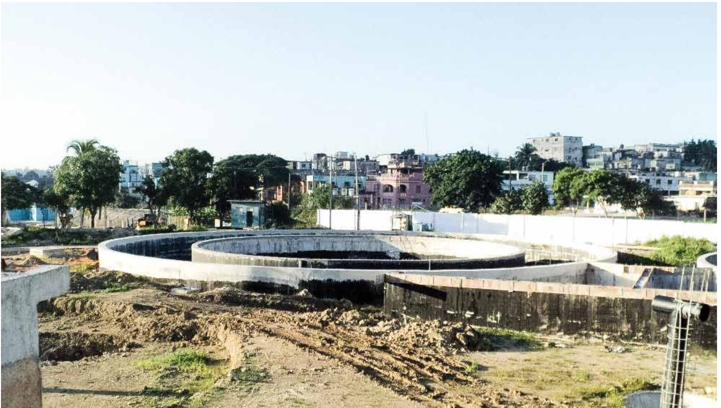
Nutrient removal reactors under construction for Havana Bay wastewater treatment facility.
