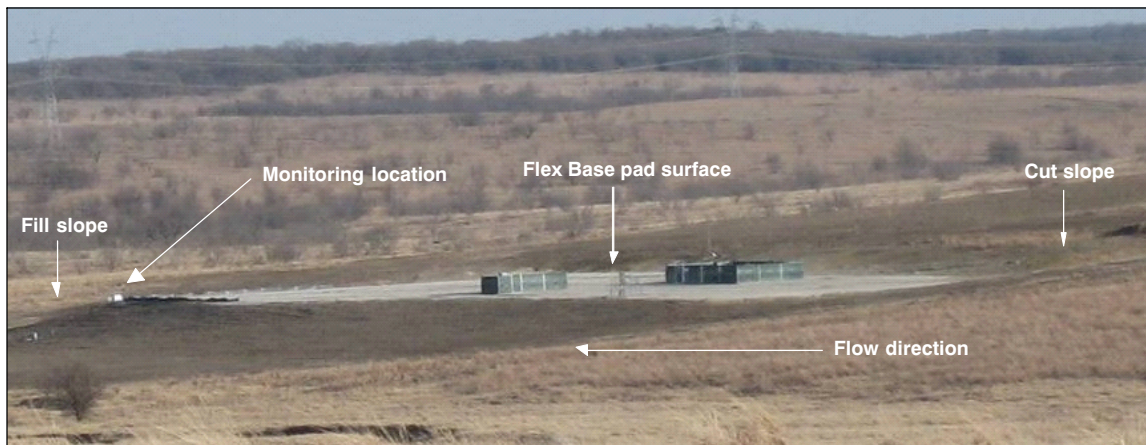
Figure 1. Gas well pad surface (GW1) on modified hillslope.
