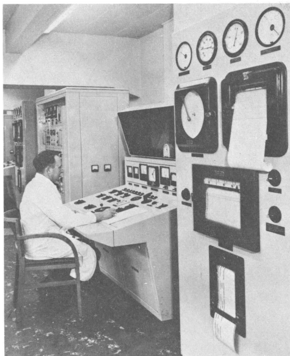
Figure 13.—Operating consoles for vacuum arc furnaces in the Kynoch works of Imperial Metals Industries, Ltd., Birmingham, England.
