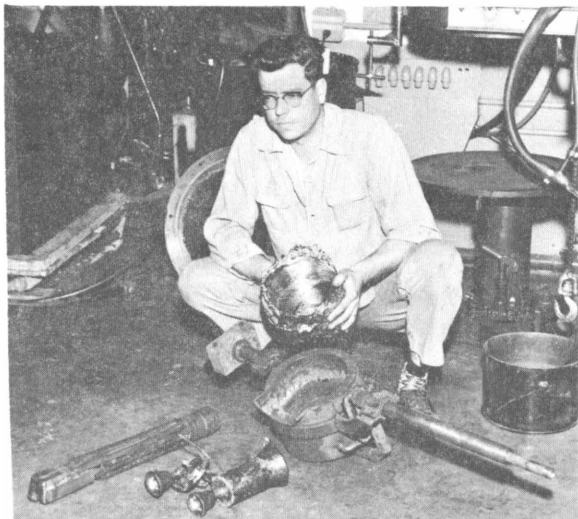
Figure 89.—Tilting crucible and skull.
