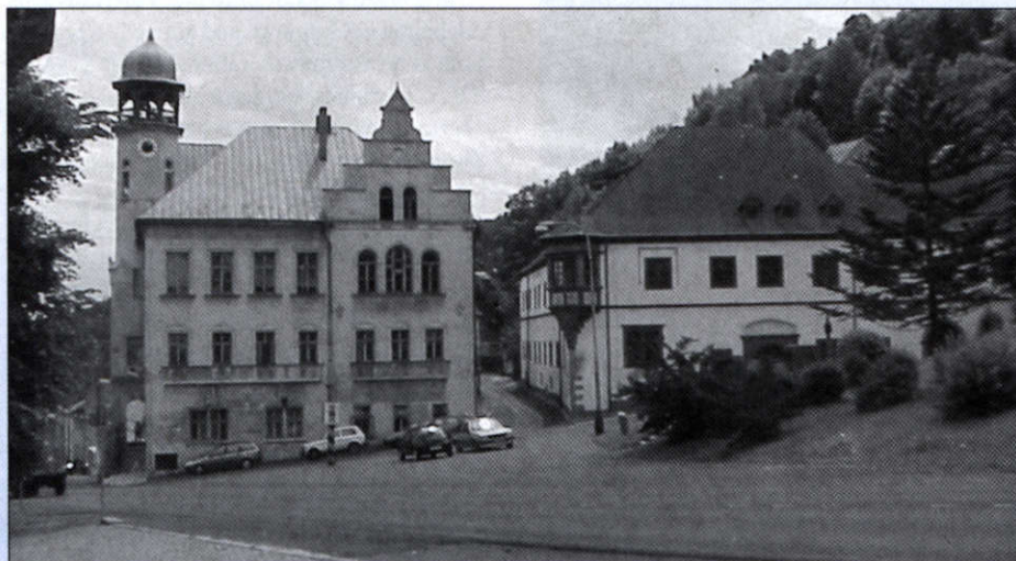
Figure 4. Jáchymov, located on the Czech side of the Erzgebirge (Krušné Hory) mountain range 5 km south of Germany, was once known as Joachimsthal, Bohemia. The two buildings are the city hall (left, which now houses the tourist bureau/museum) and the old mint (right, which dates from 1536). (Note 1).
