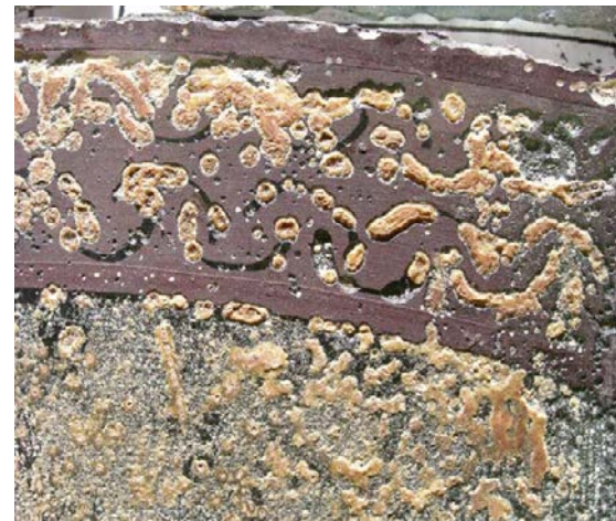
The corrosion increases the specific surface
