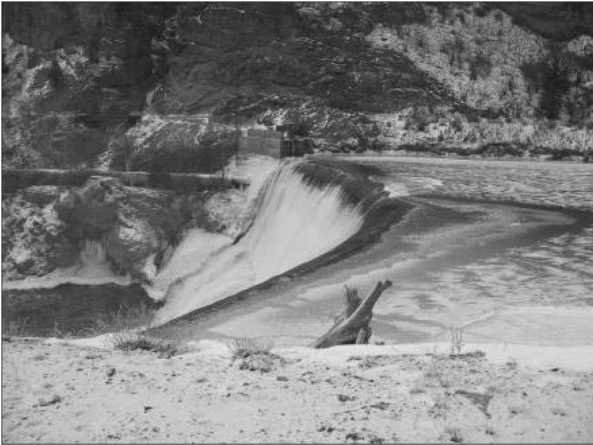
Figure 14. KOP 4, overlook near Enloe dam (Source: Okanogan PUD, 2008a).
