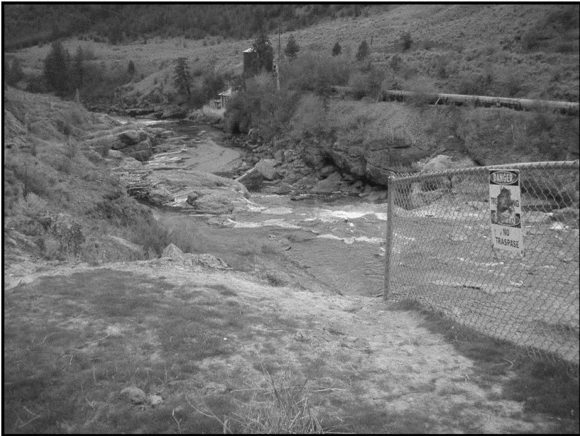
Figure 15. KOP 5, overlook east of Enloe dam, looking south (Source: Okanogan PUD, 2009h).
