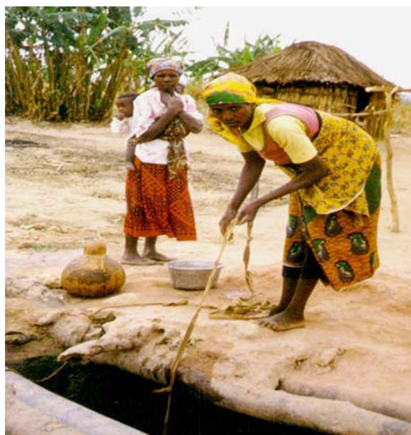
Figure 5. Wood employment in a hand drilled well in Zambia (Sutton 2002).
