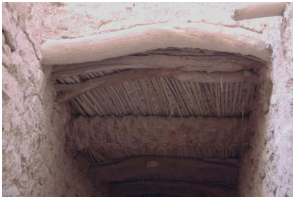
Figure 4. Covering system made of half date palm trunk, tamarisk beams and date palm midribs (Al-'Ula, Saudi Arabia, © C. Bouchaud).
