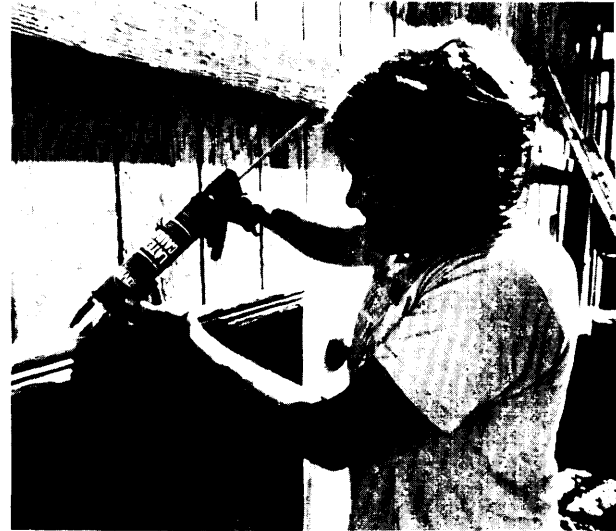
Photo credit: U.S. Department of Energy
