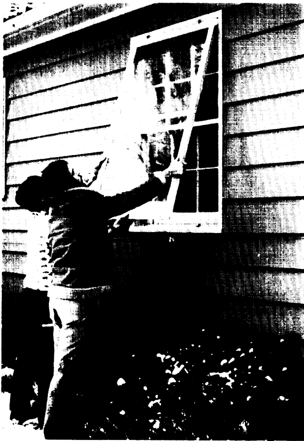
Photo credit: U.S. Department of Energy
