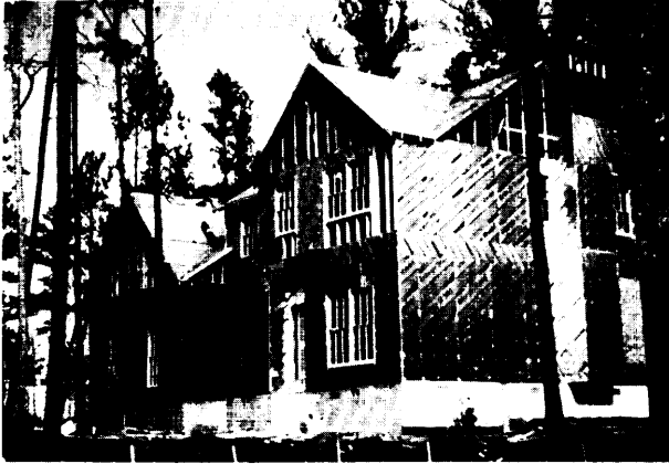
Photo credit: Electric Power Research Institute
