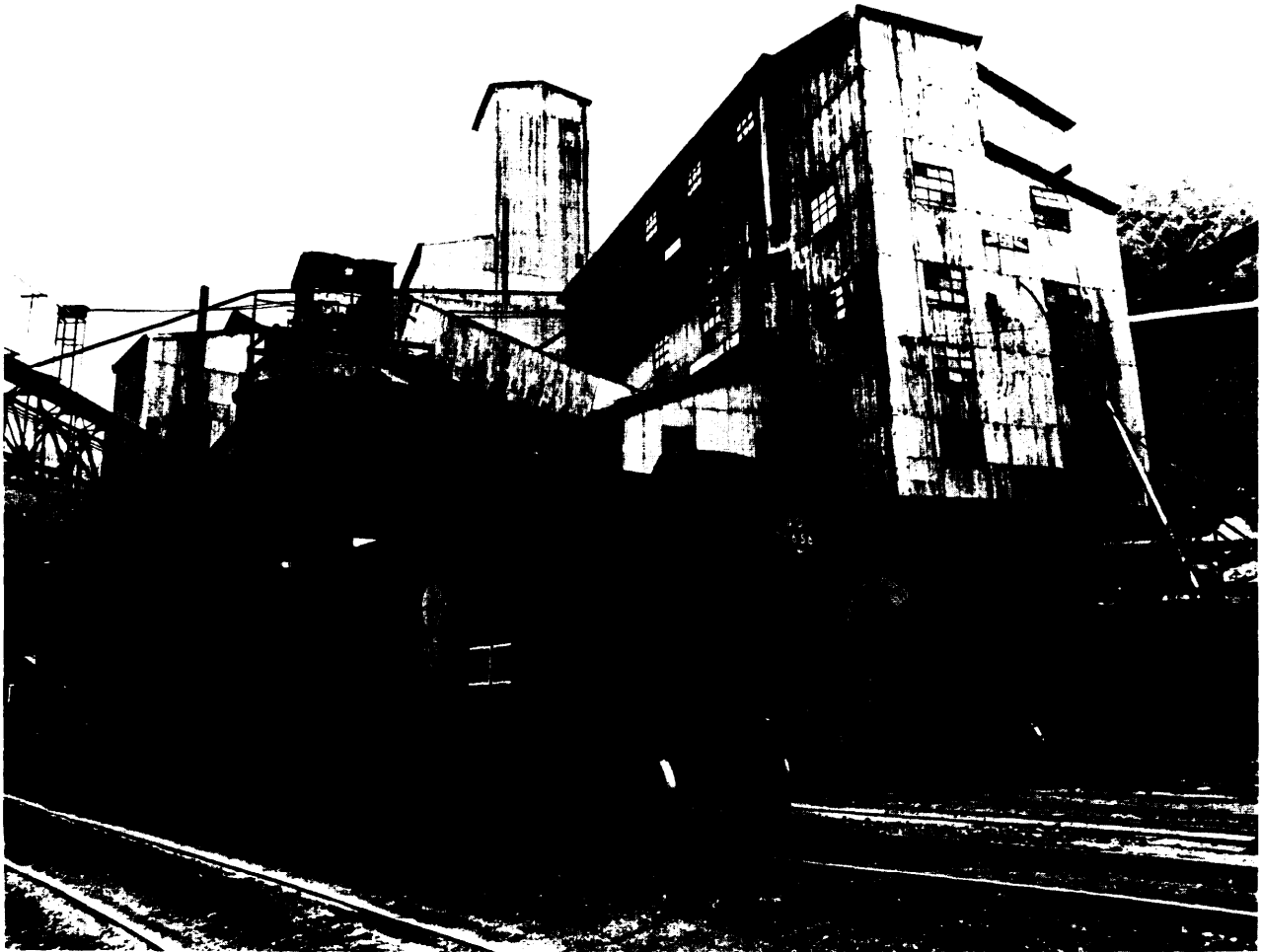
Coal tippie on Cabin Creek, W. Va.
