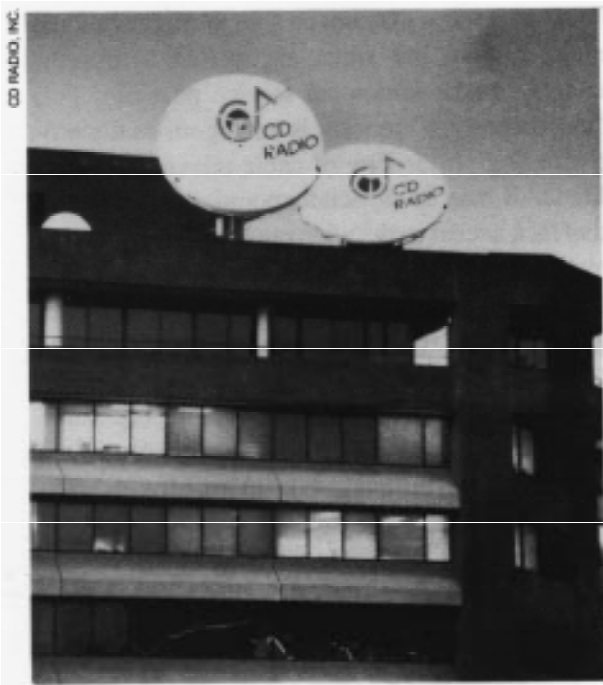
Satellite dishes such as these will beam digital quality radio programming up to satellites that will then retransmit it across the country
