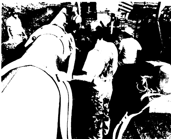
FIGURE B-3: Pipeline Rehabilitation
