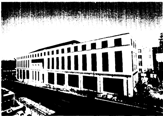
FIGURE 1-5: The National Climatic Data Center Building, Asheville, North Carolina
