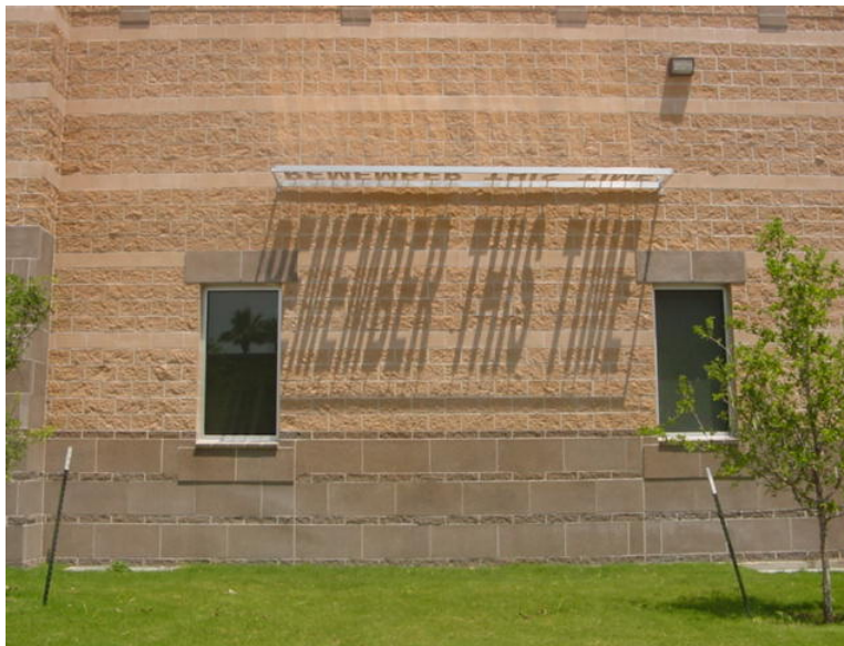
Figure 4.16. Remember This Time, fall 2005 semester program public art product. as photographed on May 5, 2006, shortly after its installation.
