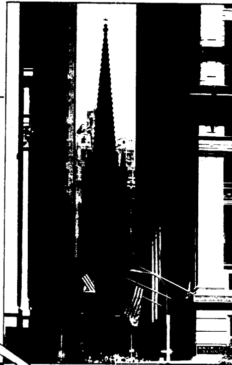
Trinity Church (located on Wall Street in Manhattan). The church appears black in the photo, due to many years exposure to soot. Recent cleaning restored the church's stone to its original pinkish color.
