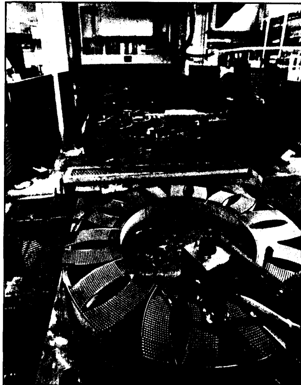
FIGURE 3-13: RECUPERATOR MANUFACTURING FACILITY
