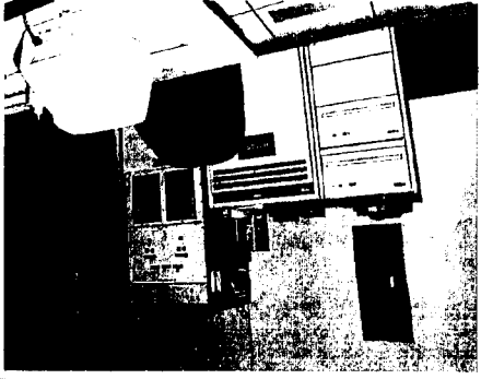
WCS Communication Facility
