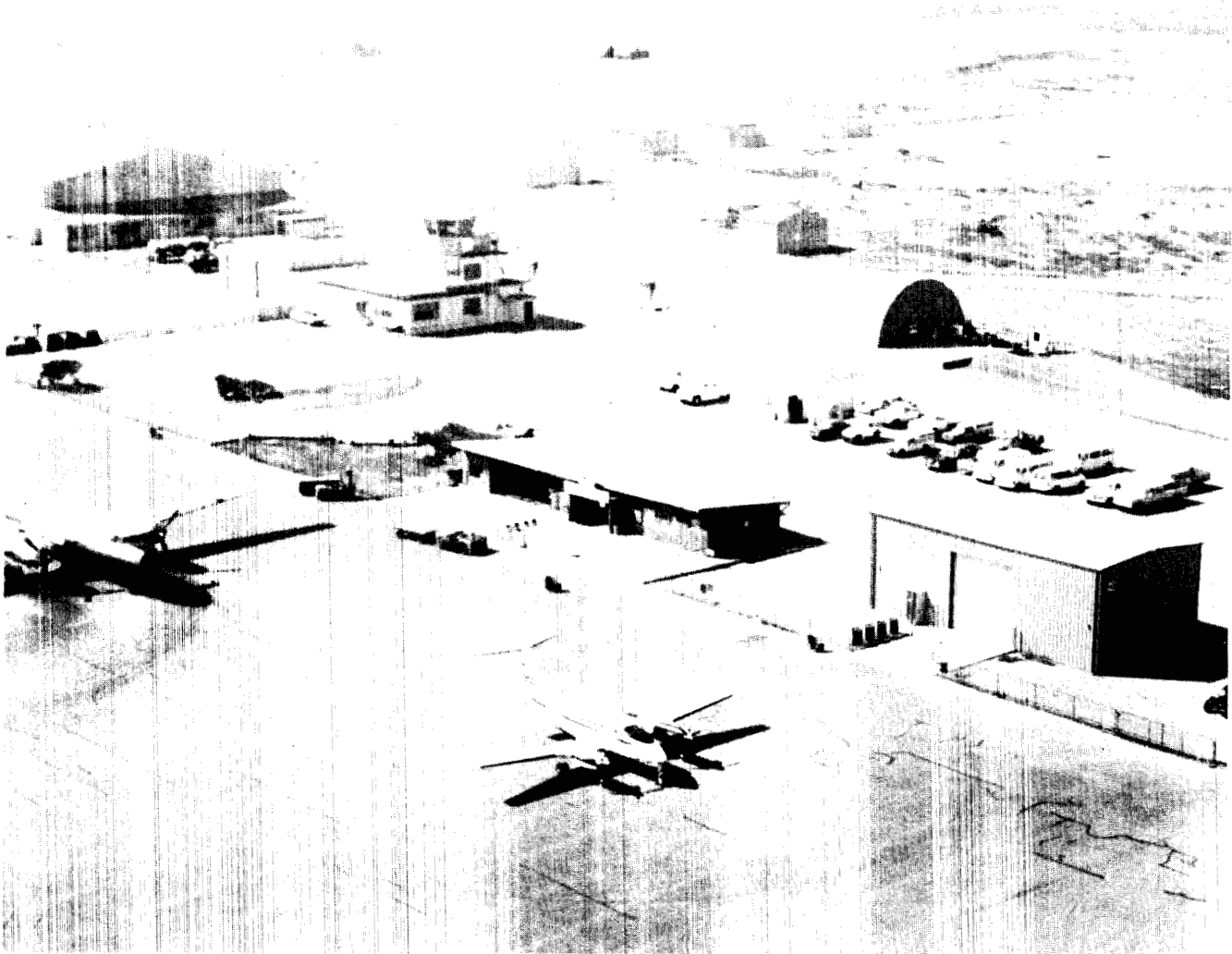
The SNI airfield, air terminal, air traffic control tower, ground support equipment storage building, aircraft target hangar, supply warehouse and hazardous waste stations are all part of the SNI airfield complex. The Convair 440 used for shuttling passengers to/from Point Mugu is also seen here with the smaller C-12 Range Operations aircraft.
