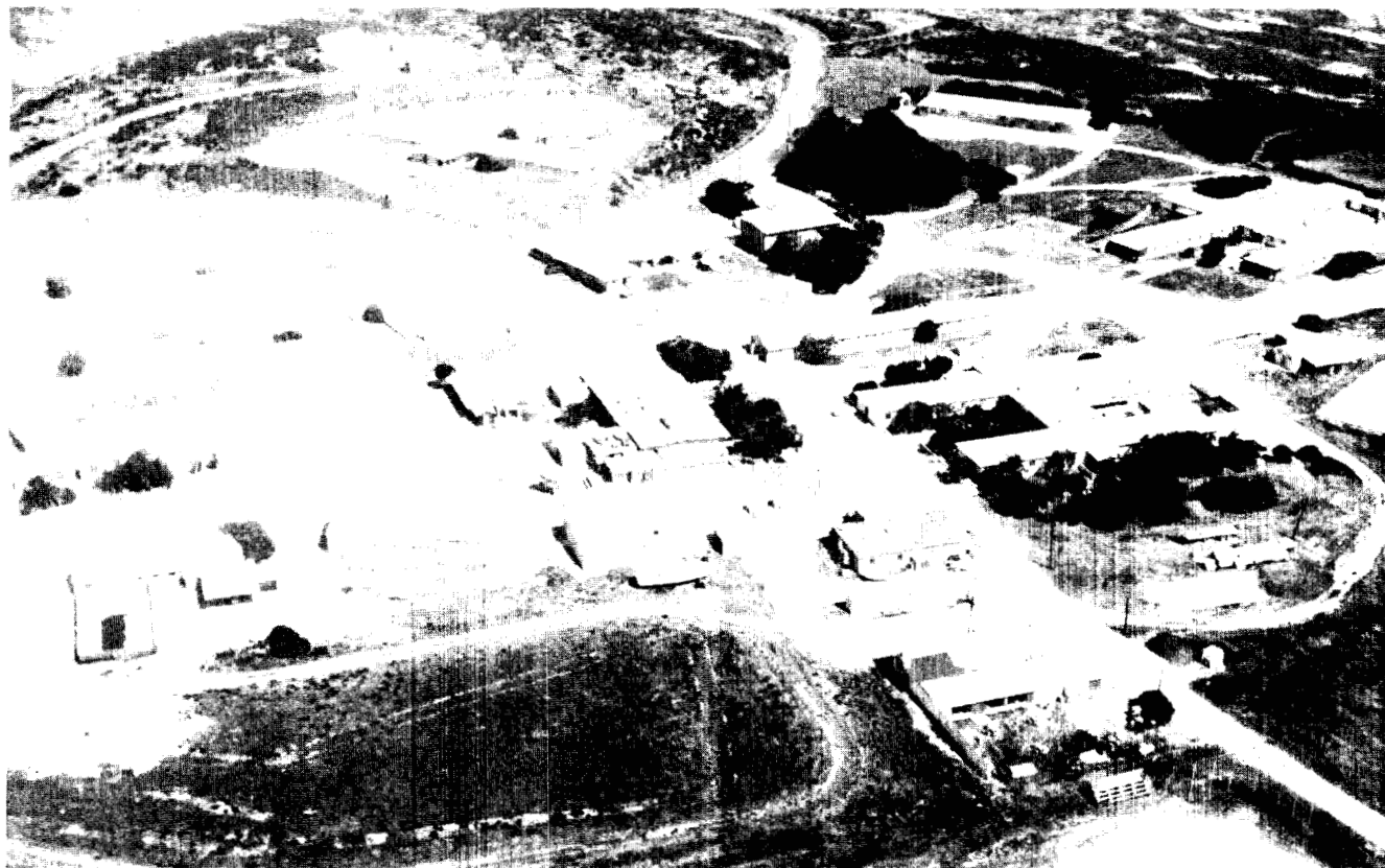
"Nicktown" is home to approximately 250 military, civilian, and contractor employees on SNI. All services and facilities are located within the compound.
