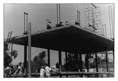
poured on it. Another day, another coat of oil, and the roof slab was poured. When all three slabs were properly cured, up went the roof and the second floor into place. The walls could then be added. The building was at this unwalled state when we held the ceremony.
