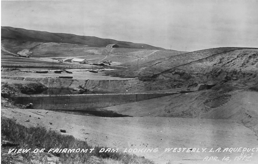
Figure 19: "View of Fairmont Dam looking westerly. L.A. Aqueduct. April 14, 1912." Special Collections, Honnold/Mudd Library, Claremont University Consortium.
