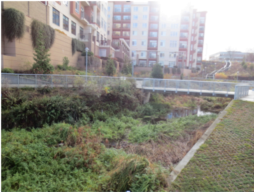
Figure 8. The Thornton Creek Water Quality Channel and surrounding high-density retirement living is publicly accessible by pathways and bridges. The Channel is also equipped for maintenance by SPU as it collects sediments. Photo by author.
