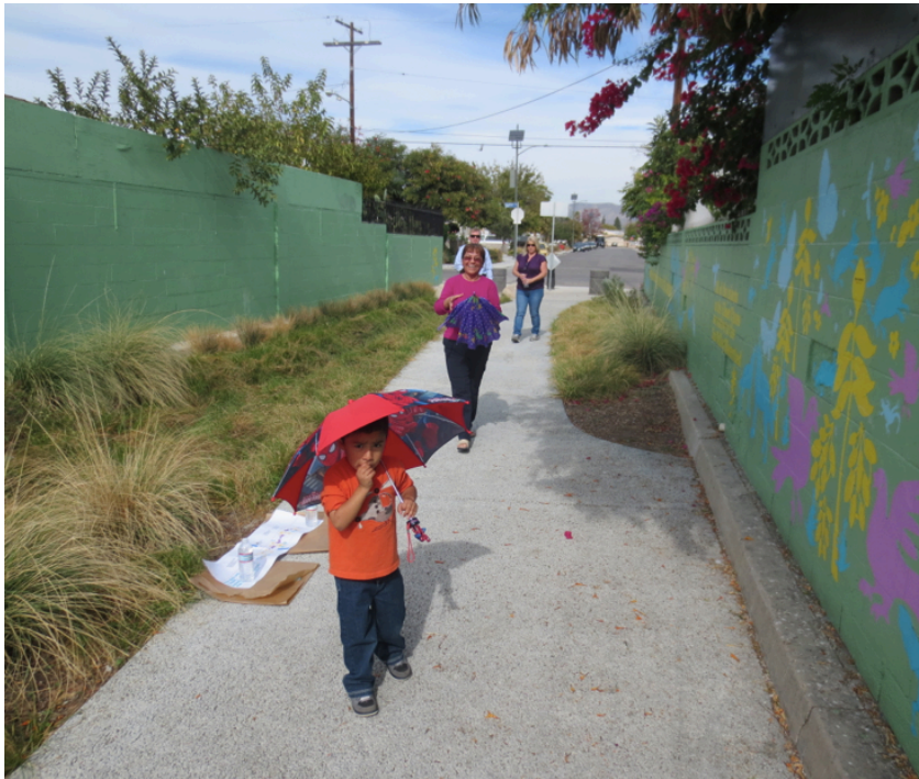
Figure 12. Residents and visitors to the Elmer Paseo walk through on the newly constructed permeable pavement path. Elmer Paseo infiltrates stormwater from 7 acres and is designed as a safe community space. Photo by author.
