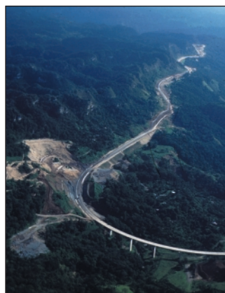
Photo 62. The transformation of the karst belt by the construction of Highway PR 10 through the Río Abajo Commonwealth Forest. The section of road in the foreground is considered among the most expensive road constructions—per kilometer—in the world. Photo by J. Colón.
