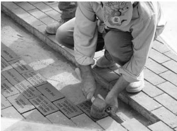
A worker in the process of laying the first 100 bricks.
