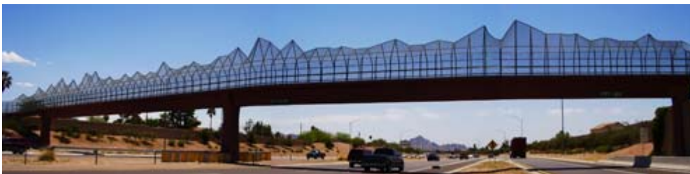
Figure 7: Mountain Pass Pedestrian Bridge. Source: Laurie Lundquist
