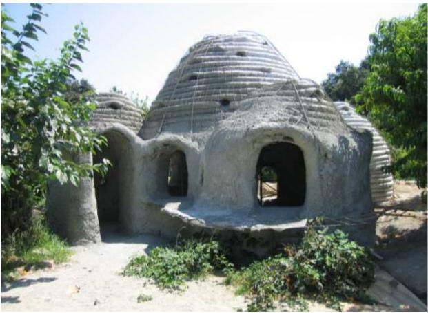
Figure 3: The second Earth Dome at the Pomona College Organic Farm in July 2005. Note the tubes of soil, the rebar and wire mesh, and the first layer of gunite on the bottom half of the structure. *http://en.wikipedia.org/wiki/File:Front\_of\_dome.jpg*.
