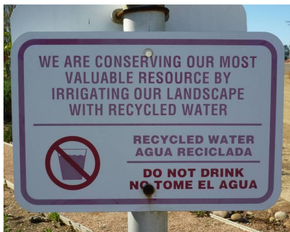
Required signage to mark non-potable reuse
