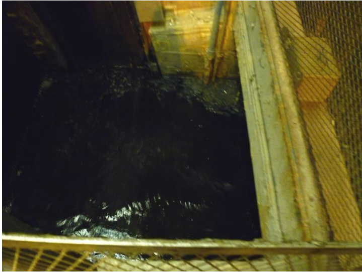
Initial filtration designed to remove rags, sticks, rocks, and any relatively large items.
