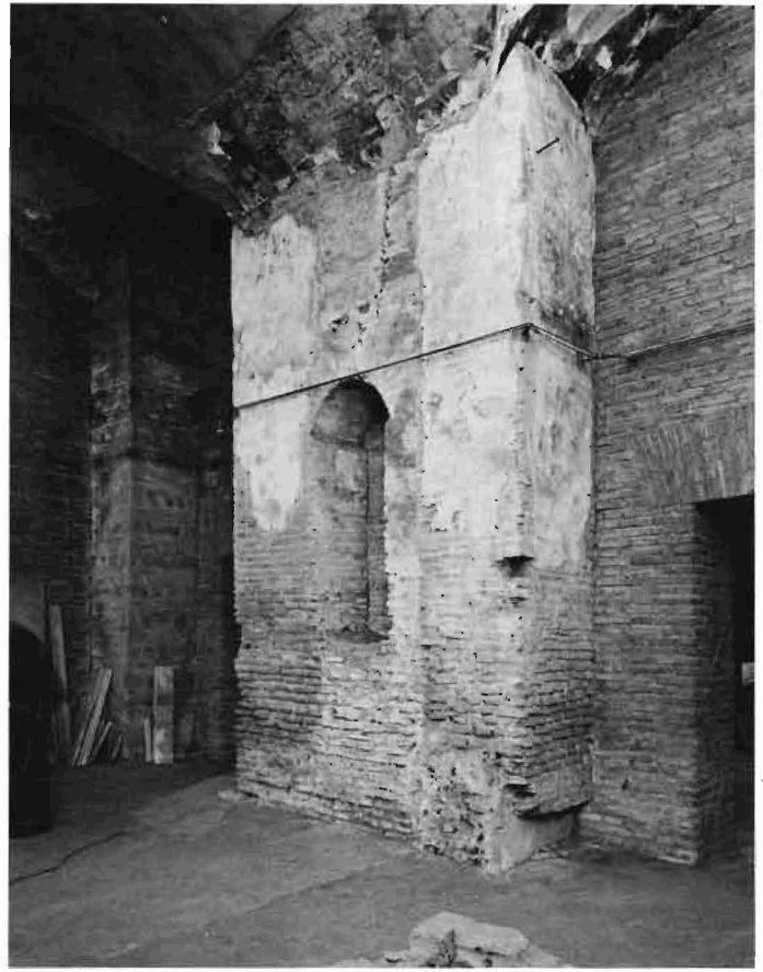
18. View of Pier One from the South West
