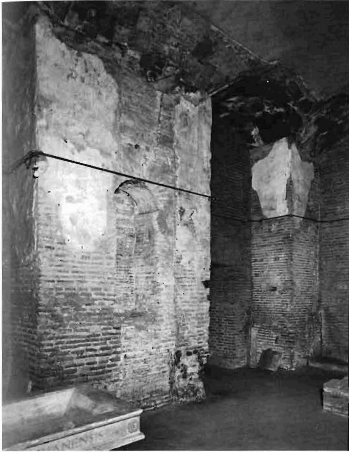
17. View of Piers One and Two from the North West
