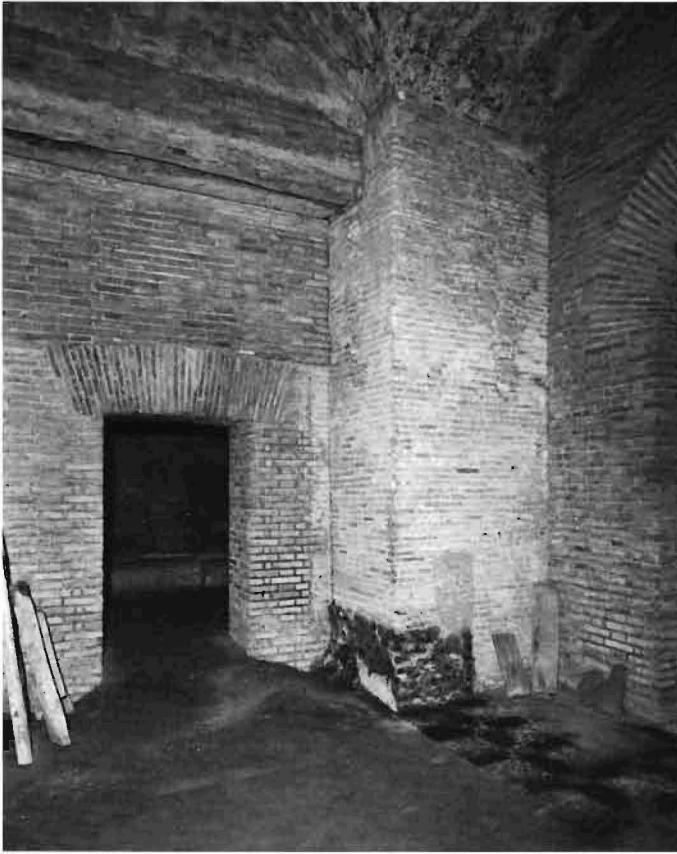
23. View of Pier Four from the North West in Room H
