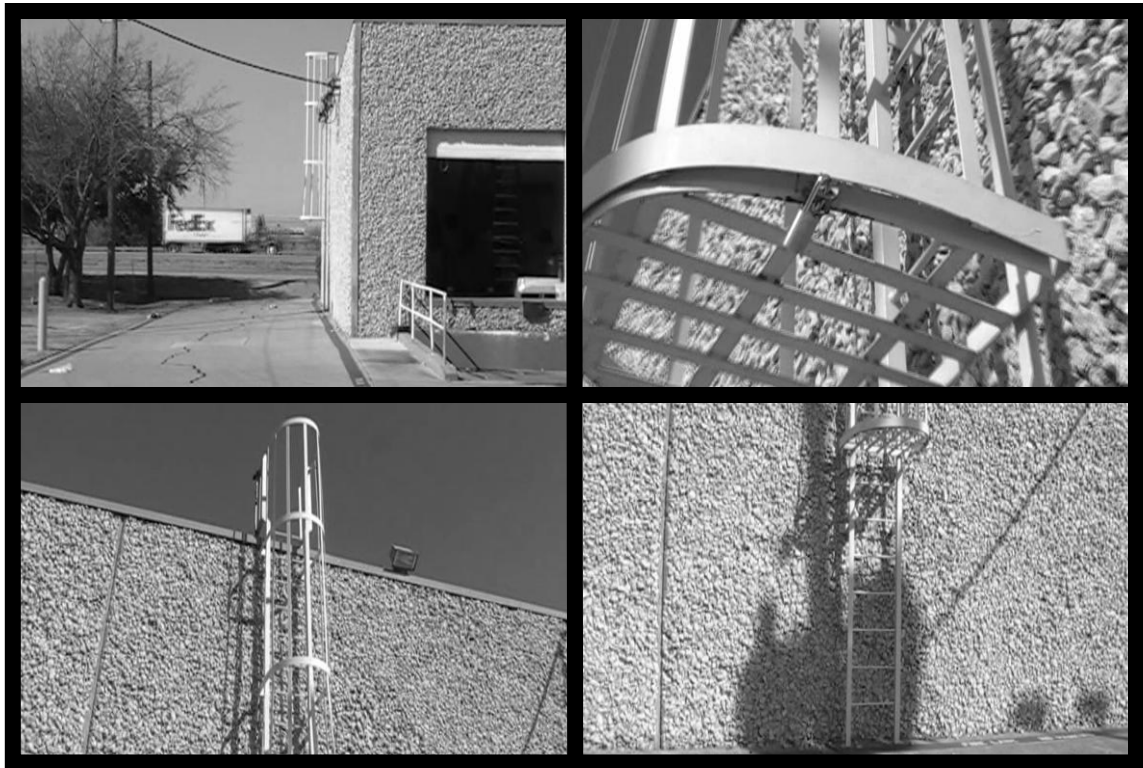
Figure 6. The building owner had locked this ladder cage. The customer did not have a key. The Metro Environmental 30-foot ladder would not reach the roof. The technicians decided to climb the building on the outside of the ladder cage. They carried parts, tools, and the SightPros communication tool to and from the roof.
