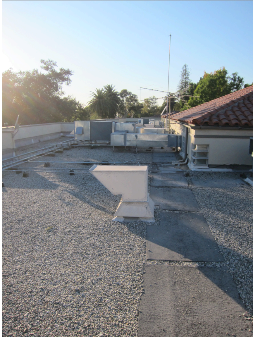
(Fig 20) On Lyon Hall there is another gravel roof. (12/6/11)
