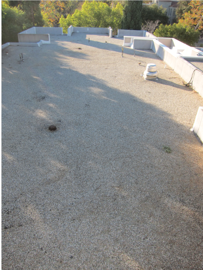
(Fig 18) Oldenburg also sports a gravel roof, with a small area covered with a reflective coating. Oldenburg is a low profile building with one of the most expansive flat roofs on campus, and so is a location that should be considered for a reflective coating. (12/6/11)
