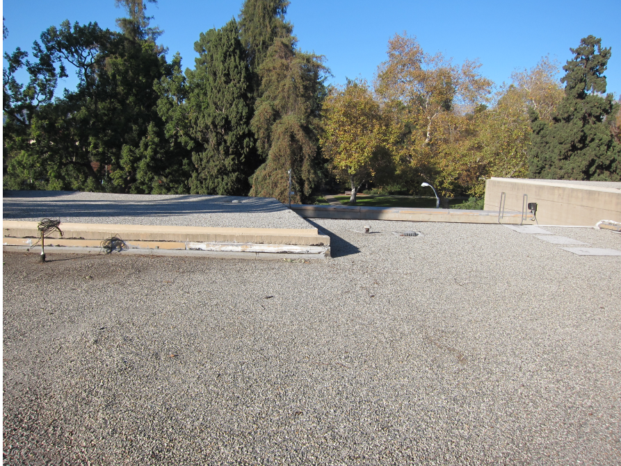
(Fig 14) This is the roof on top of the Thatcher music building. This is a very common inexpensive roof where asphalt, bitumen, and felt are laid over a concrete slab and then gravel is spread over the top. (12/6/11)
