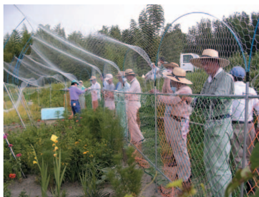
Fence to prevent intrusion by monkeys or wild boars (Installing “ Oumi Enraku/Shishi Dome Kun ” fence)
