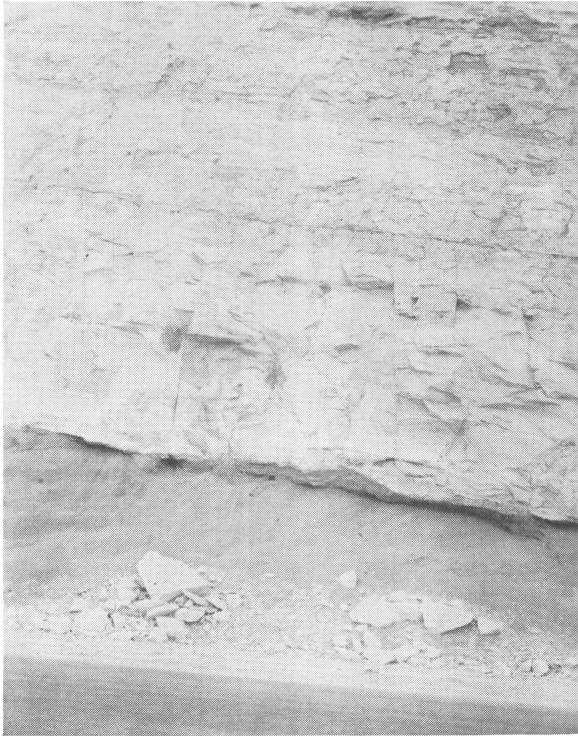
FIGURE 22.—California 4 deposit, Shasta County. Note ash and thin alluvial-material stratum.
