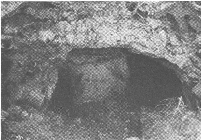
FIGURE 10.—Entrance to abandoned workings at Washington 1 deposit.
