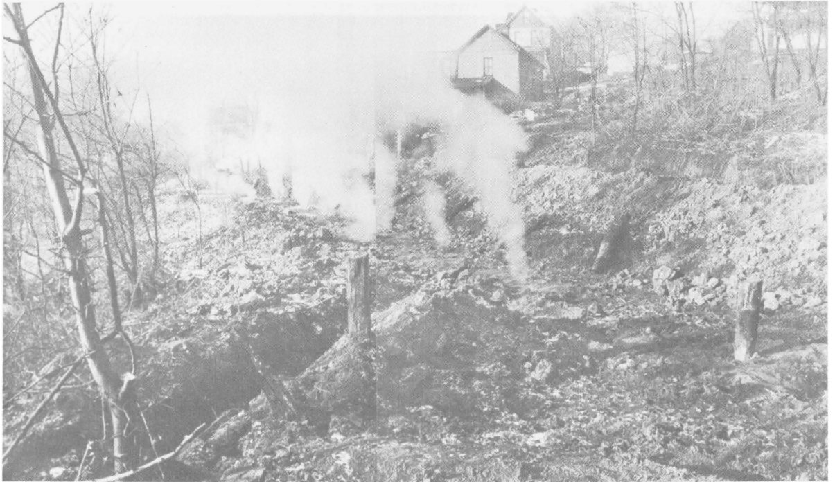
FIGURE 22.—Smoke and Steam Issuing From Boreholes Before Flushing With Incombustible Materials. Drilling Operations in Background.
