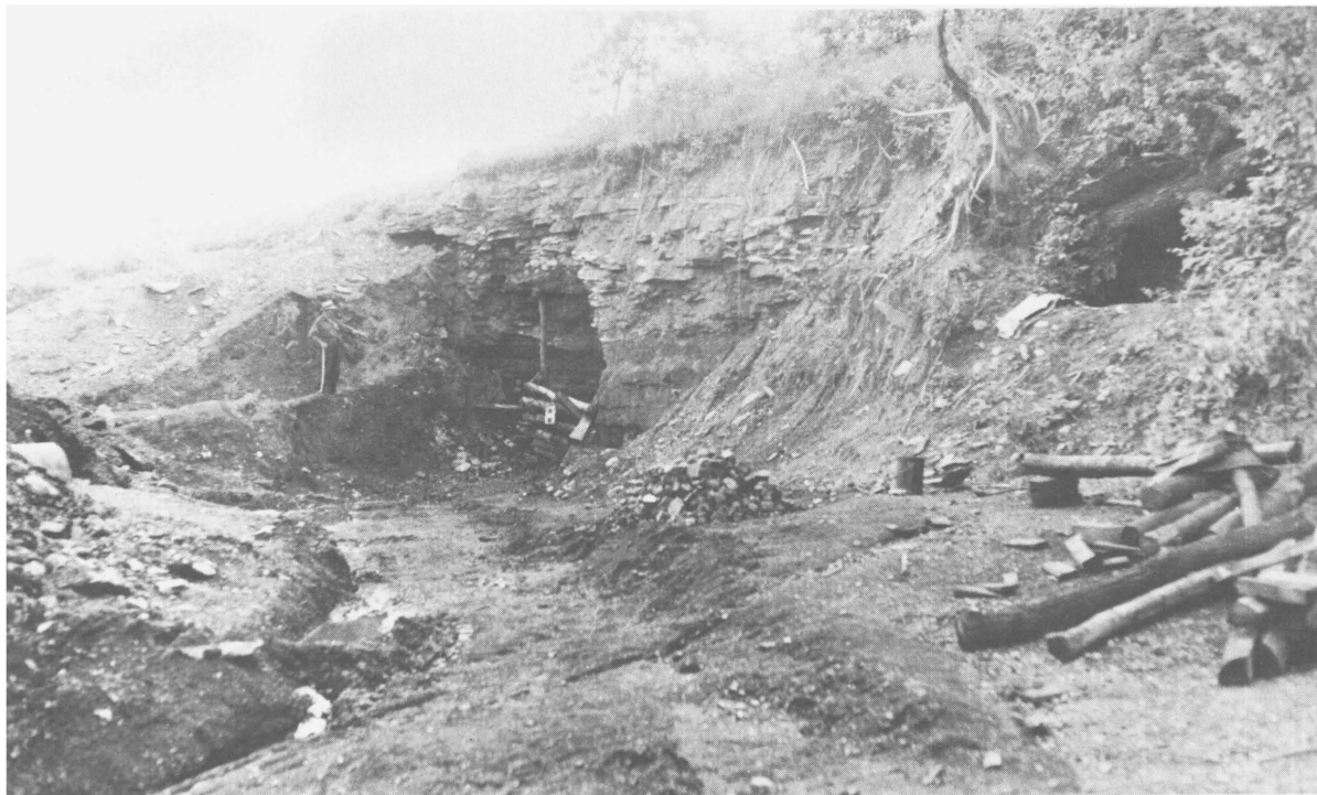
FIGURE 5.—Site Where Burning Coal Was Stripped Along Outcrop and Abandoned Portal of Mine, Monessen City Park Project.
