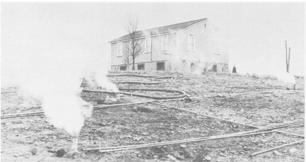
FIGURE 60.—Site of First Experiment. (Some boreholes purposely uncapped to show steam issuing from underground fire.)
