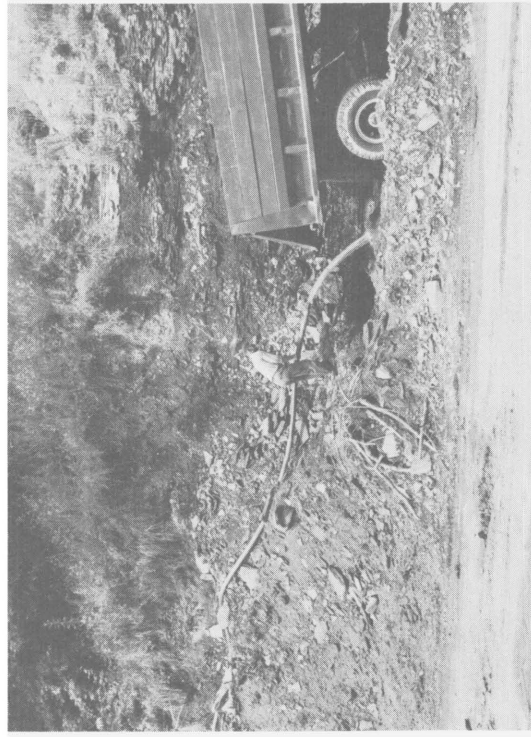
FIGURE 19.—Several Operations Employed in Drilling and Flushing Underground Openings Along Legislative Route 118 Near Pricedale, Pa.
