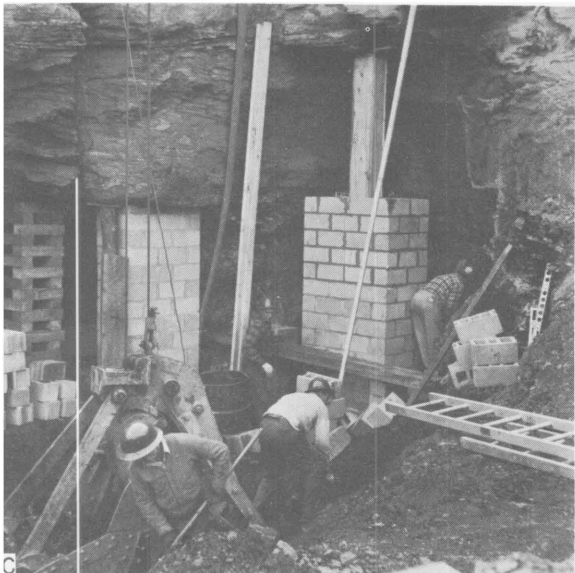
FIGURE 8.—Cooling Materials Before Loading-Out Operation; B , Clamshell Loading-Out Blasted and Cooled Material; C , Installing Masonry and Wooden Supports Before Backfilling; D , Backfilling Excavated Fire Area; E (p. 26), Shoring Wall Installed to Retain Earth-Blanket Backfill; F , Completed Project, Showing Drainways and Backfilled Area.
