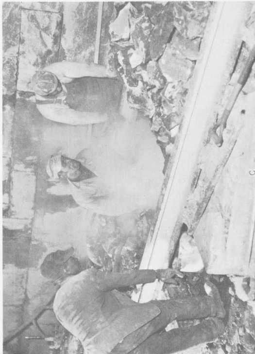
FIGURE 58.—Railroad-Tunnel Fire-Control Project: A, Opening in Stone Sidewall From Which Hot Vapors and Gases Evolved; B, Grouting Pipes Through Which Slurry Was Pumped Under Floor of Tunnel; C, Drilling Grouting Boreholes in Floor of Tunnel; D, Some of Equipment Used for Flushing Voids in Fire Area.
