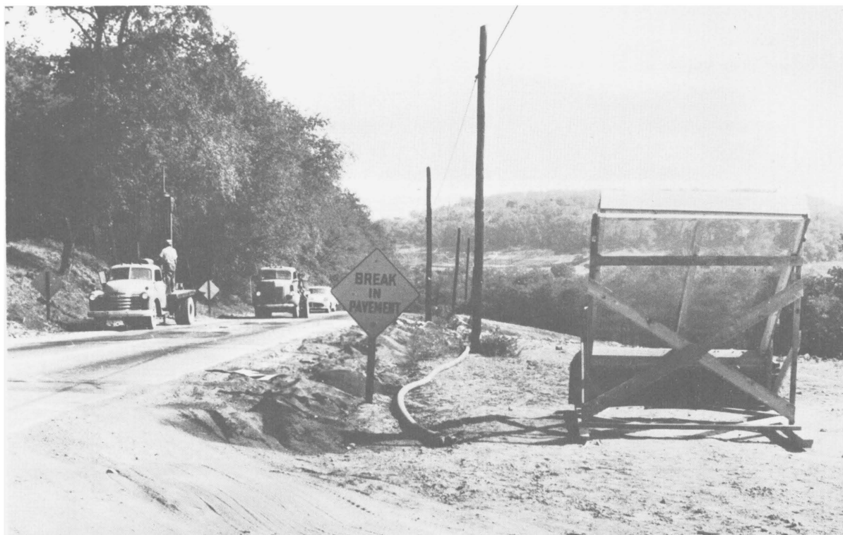
FIGURE 18.—Drilling Boreholes Along Highway in Affected Area.
