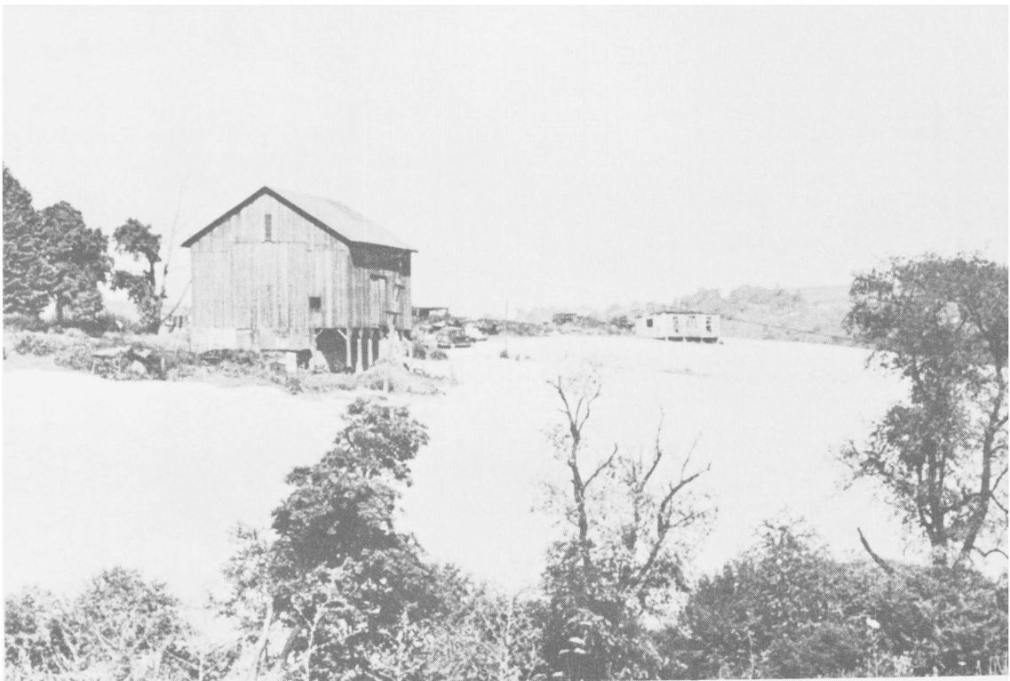
FIGURE 41.—Part of Lick Run Project Before and After Placing Surface Seal.
