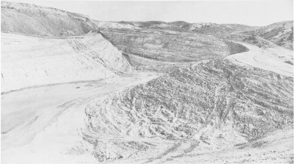
FIGURE 38.—Borrowed Fill Surface-Sealing Project as It Nears Completion. (East and south sections are completed; terracing on north wall (left) is two-thirds complete.)
