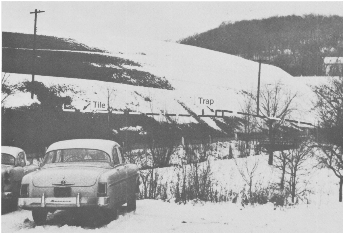
FIGURE 29.—Airtrap Drain Underlying Surface Seal at Coal Outcrop. (Dotted line traces approximate course of pipe; note how subterranean heat melted snow at left.)
