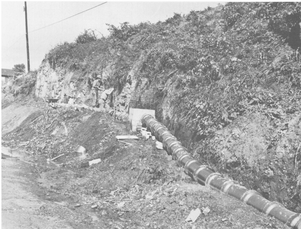
FIGURE 28.—Installation of Airtrap To Receive Drainage From Several Locations.
