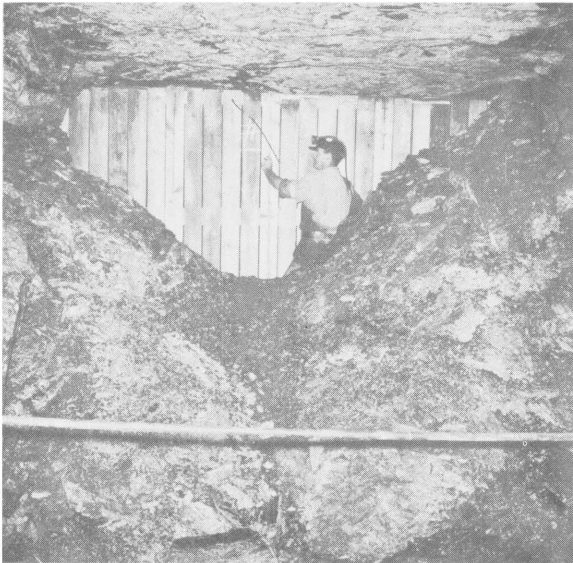
FIGURE 45.—Fire-Seal Stoppings at Various Stages of Construction.
