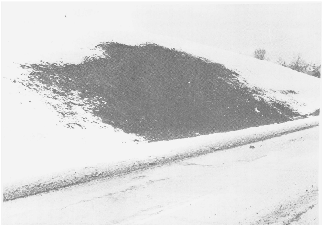
FIGURE 37.—Melting Snow Gives Evidence of Heat From Fire Area Underneath Highway.
