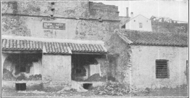
A. ORIGINAL BUSTAMENTE FURNACE BUILT AT ALMADEN, SPAIN, IN 1646 AND STILL OPERATING
