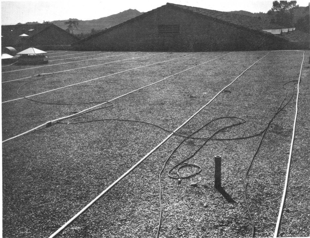
Fig. 2.25—Tubing placement on roof of North Hollywood High School classroom structure.
