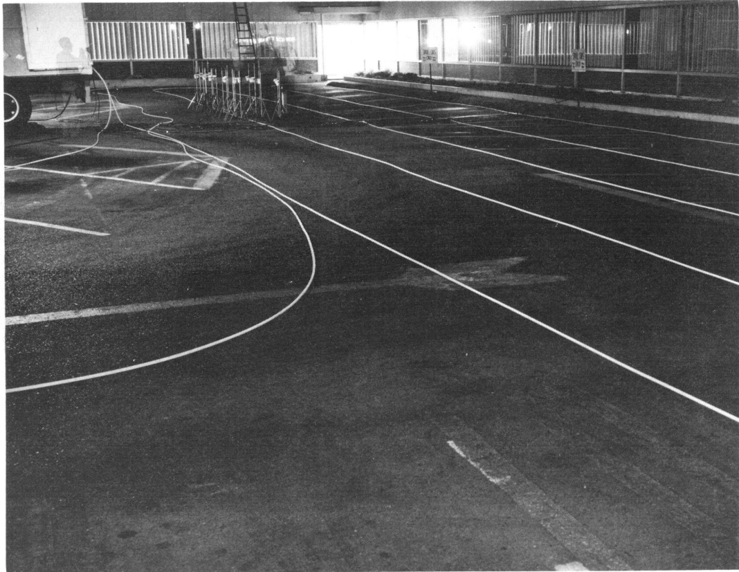
Fig. 2.24—Tubing placement on parking lot at Los Angeles Police Department building.
