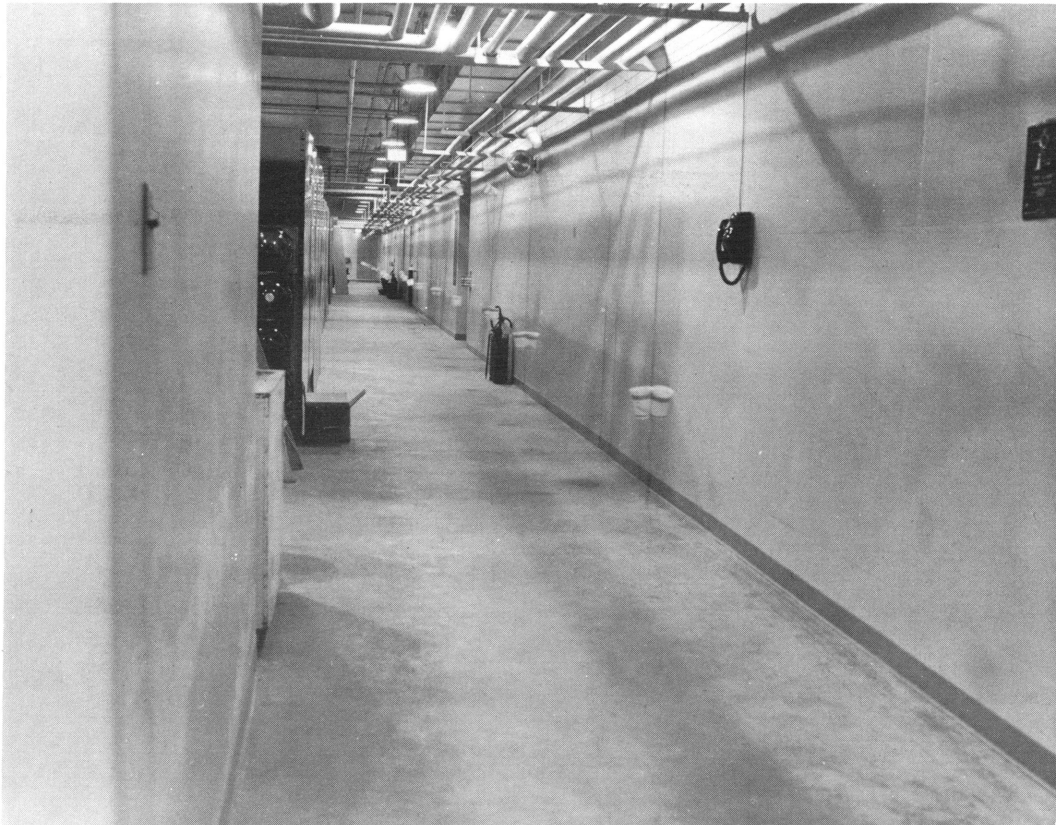
Fig. 2.18—Detector positions in basement hallway of UCLA structure.
