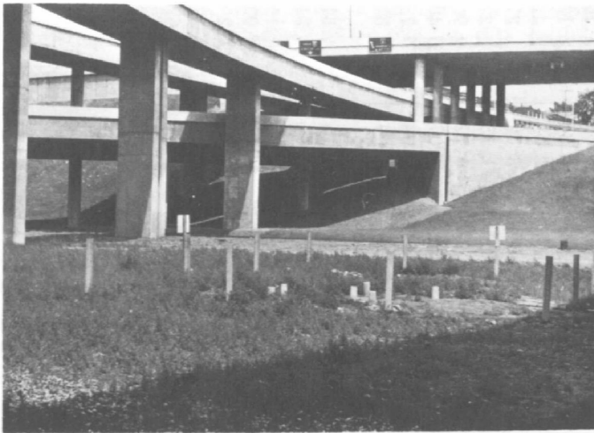
FIGURE 3. Site C—Showing surrounding highway structures.
