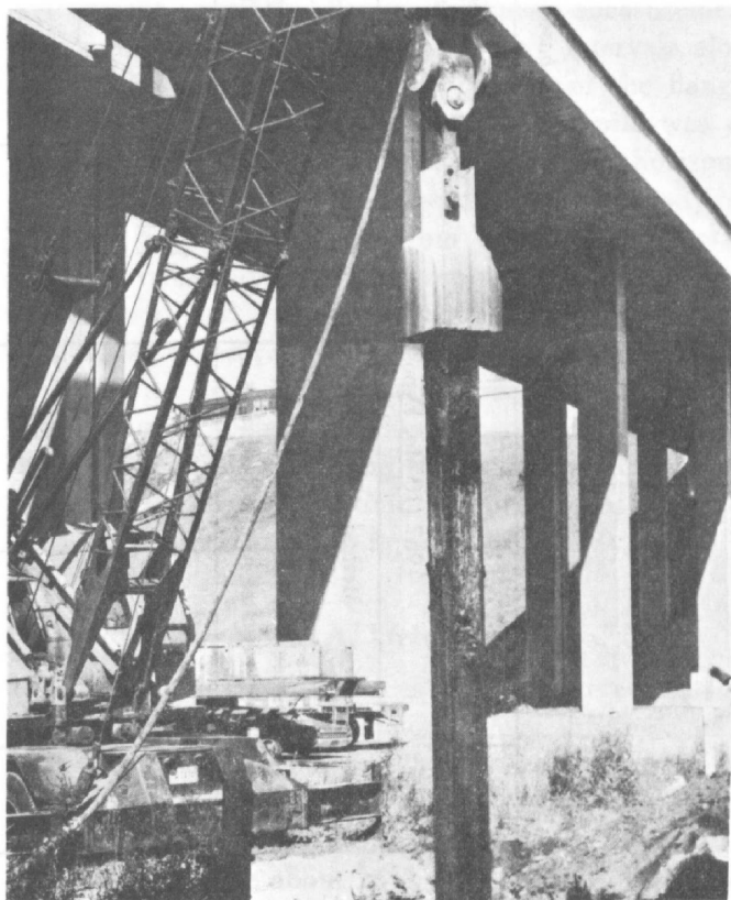
FIGURE 8. Site C—pile C1 in the process of being extracted.
