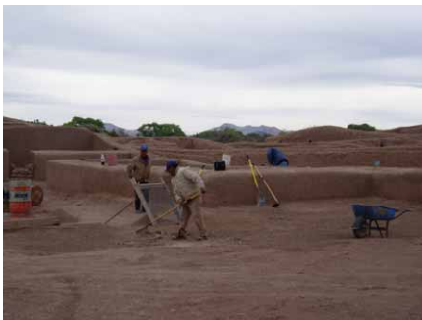
*Figure 3. Workers re-putting the adobe in March 2005. Reproduced with permission of the National Institute of Anthropology and History (INAH). CONACULTA-INAH-MEX
