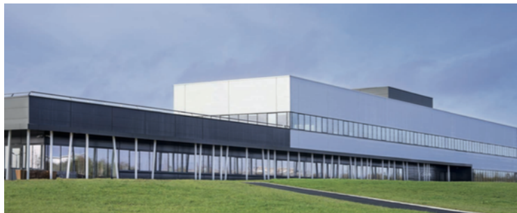
Figure 30 - La Ruche Plant In Chartres, France
