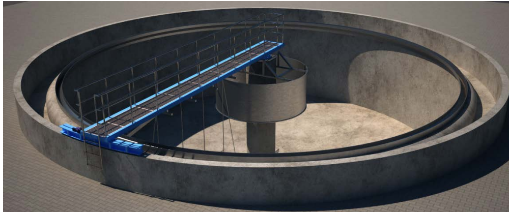
Figure 2: Secondary clarifier
